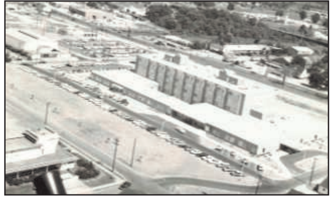
Maxwell Hospital: 1965-2000, Photo courtesy of the Air University History Office, Maxwell AFB, AL.
