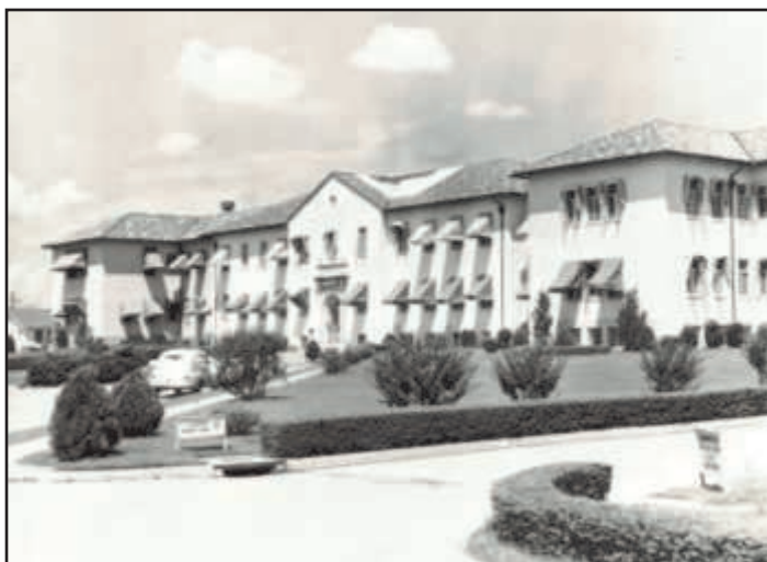
Maxwell Hospital: 1931-1965, Photo courtesy of the Air University History Office, Maxwell AFB, AL.
